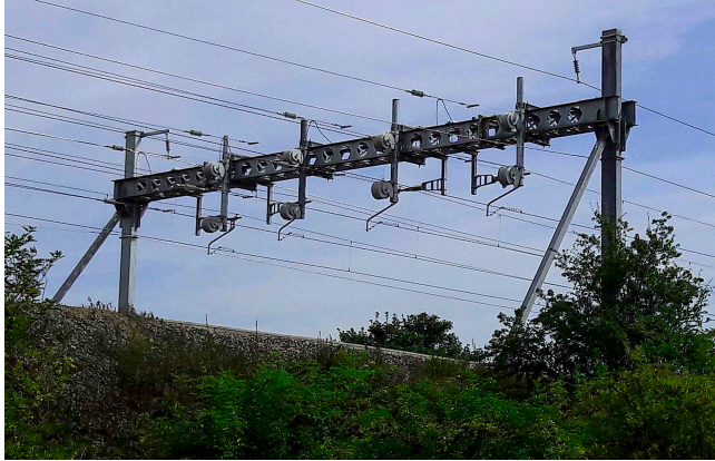
Current tension portal to support 4 single electrified wires. Photo Ian Haslam
